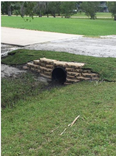
Figure 9. Driveway Culvert Installation
